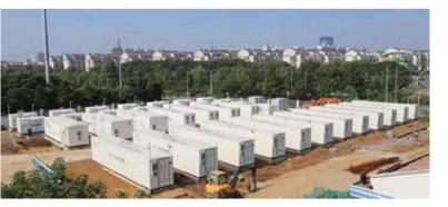
capacity is 120 MW h. The system is composed of 24 containers accommodating 400 thousand Lithium-ion batteries (Samsung SDI) assembled into 20 thousand modules.
