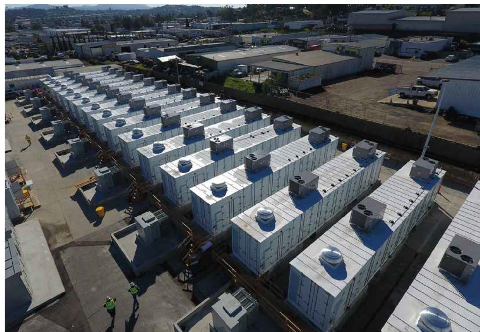
Fig. 3. 30-MW energy storage system in San Diego with a capacity of 120 MWh
