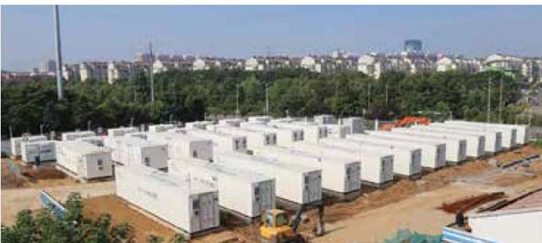
capacity is 120 MW h. The system is composed of 24 containers accommodating 400 thousand Lithium-ion batteries (Samsung SDI) assembled into 20 thousand modules.
